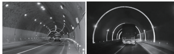
图1 隧道反光环和反光条有利于发现前车 Fig.1 Tunnel reflective rings and strips are beneficial for detecting vehicles ahead
