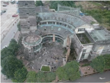
图3 社会事务服务中心大楼 Fig.3 Social affairs service center building
