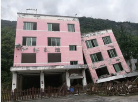
图4 消防队大楼 Fig.4 Fire brigade building
