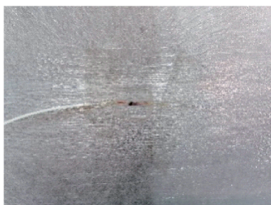
(b) 阵面安装的FBG应变传感器 (b) FBG strain sensors installed in array surface
