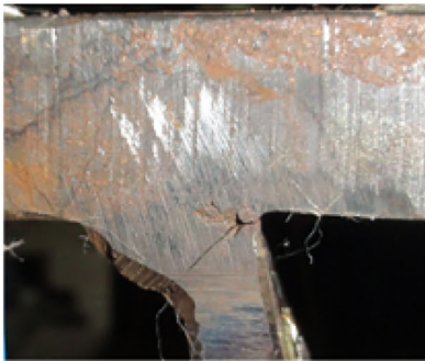
Weld penetration rate of 65% (a)
