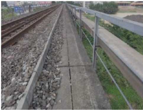
Figure 1. Railway concrete T-beam steel railings and supports. Source: Internet
