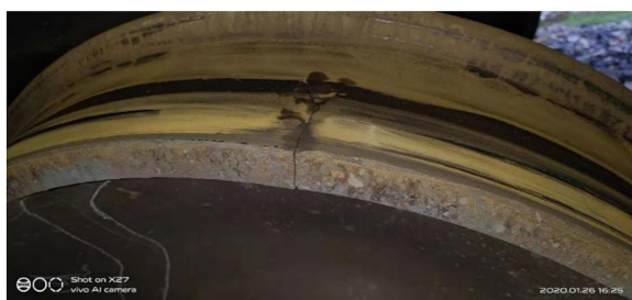
a rim crack of 28 mm
