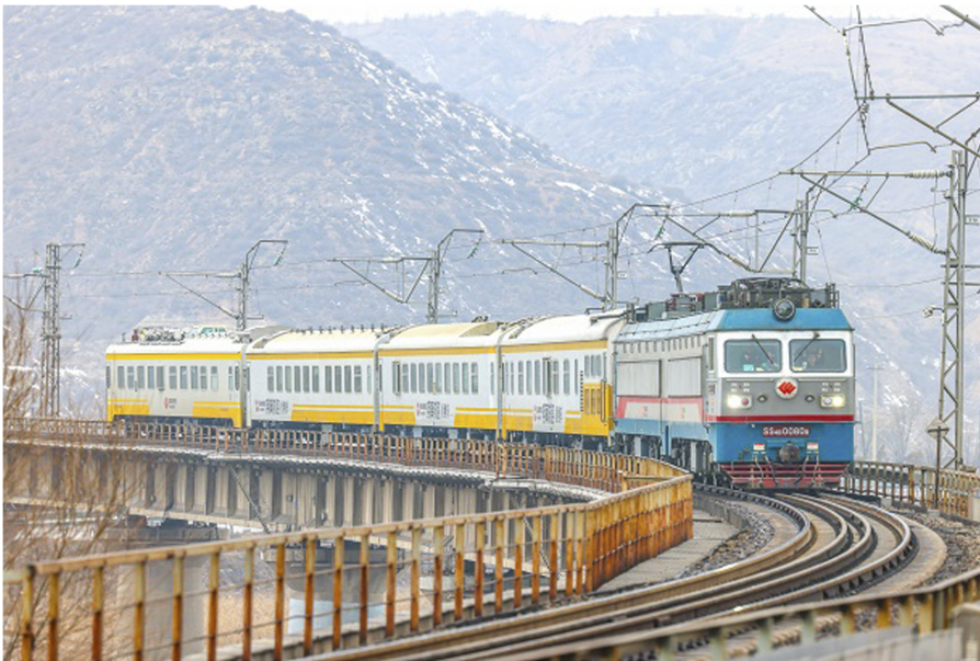
Figure 1. Heavy-haul comprehensive inspection vehicle. Source(s): Authors' own work
