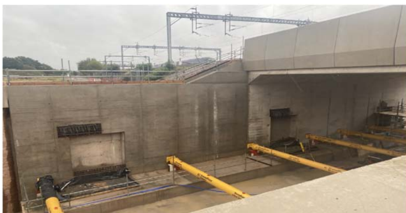
Plate 8. Fulfen Wood overbridge with temporary props in place and corbels being removed. Source(s): HS2 Ltd (2023a)
