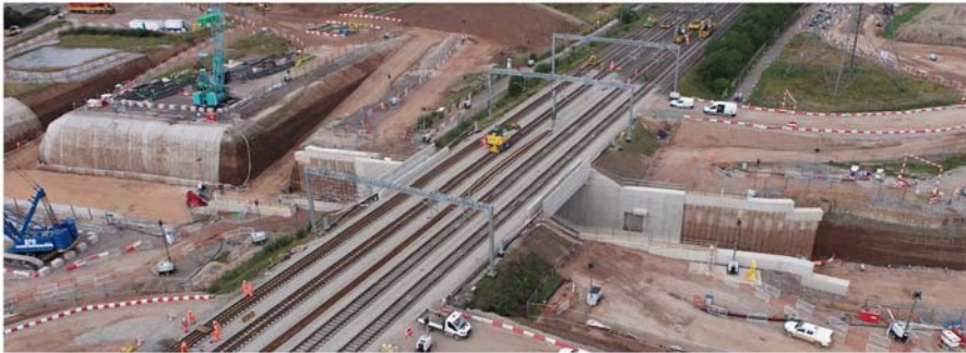
Plate 9. Fulfen Wood overbridge in position during possession and rails being replaced. Source(s): HS2 Ltd (2023a)
