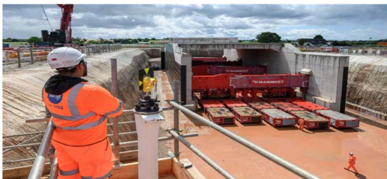
Plate 7. Fulfen Wood overbridge with SPMT lifting and positioning bridge. Source(s): HS2 Ltd (2023a)
