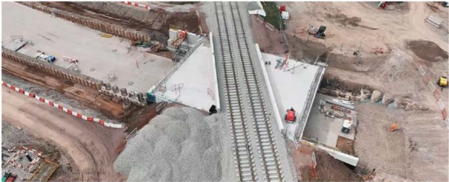
Plate 12. Streethay overbridge in position and track replaced. Source(s): HS2 Ltd (2023b)
