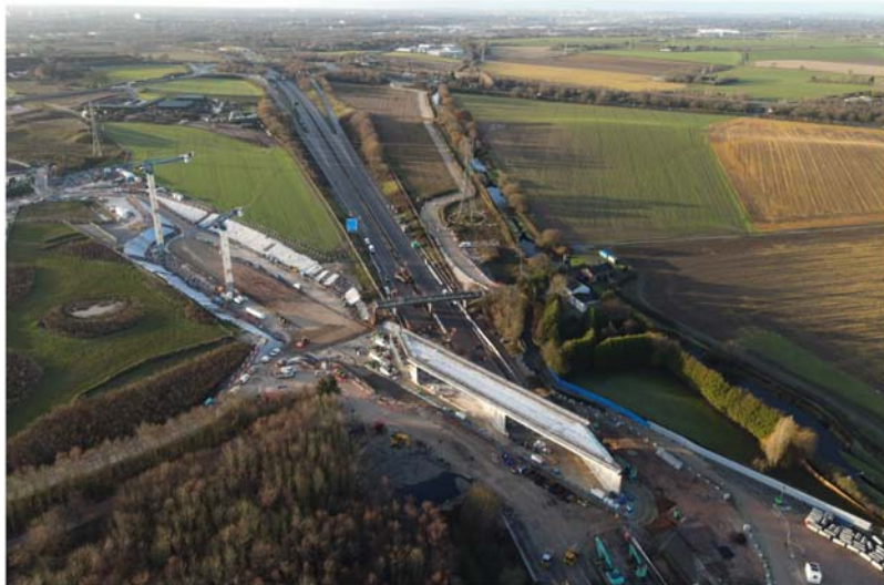
Plate 5. M42 Marston box sliding over the motorway. Source(s): HS2 Ltd (2022)
