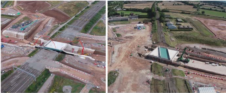
Plate 13. Fulfen Wood (left) and Streethay (right) overbridges in place during their respective possessions. Source(s): HS2 Ltd (2023a, b)
