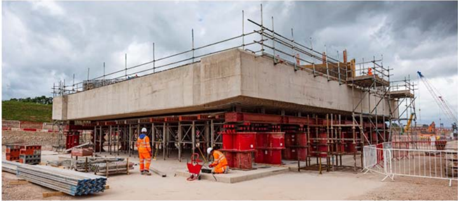
Plate 11. Streethay overbridge simply supported whilst temporary supports are removed. Source(s): HS2 Ltd (2023b)
