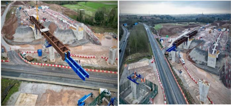
Plate 4. M42/M6 link Viaduct launch using push/pull technique. Source(s): HS2 Ltd (2024a, b, c)
