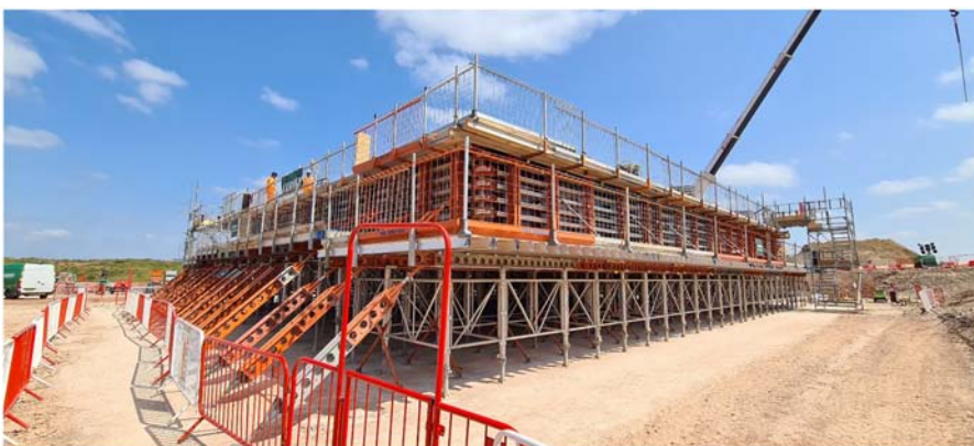
Plate 10. Streethay overbridge construction on temporary supports to allow SPMTs to lift bridge from underneath. Source(s): HS2 Ltd (2023b)
