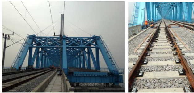
Bridge structure end view and REJs at beam end
