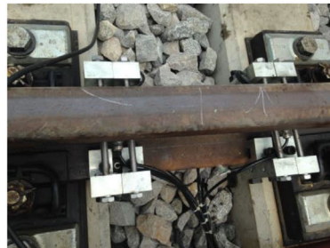
Ground inspection unit installed on track
