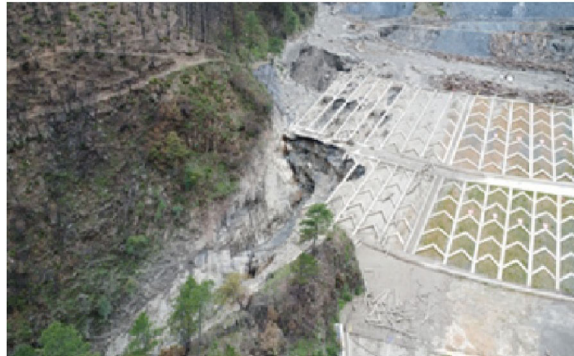
Figure 5. The slope of engineering spoil after the erosion of debris flow. Source(s): Authors' own work
