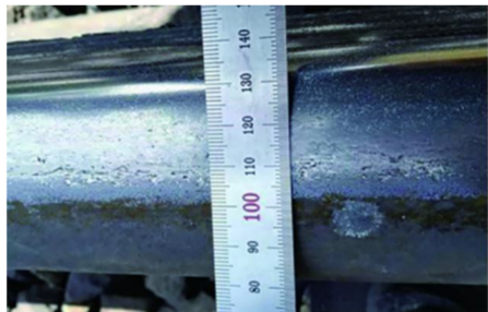
Curve section of the spiral-curve upper track at K496 of the border section of Harbin-Suifenhe Railway
