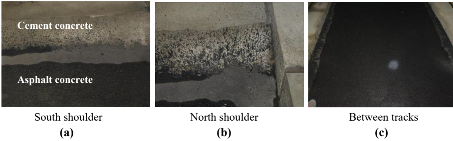
Plate 4. The overall condition of FSACWSS test section
