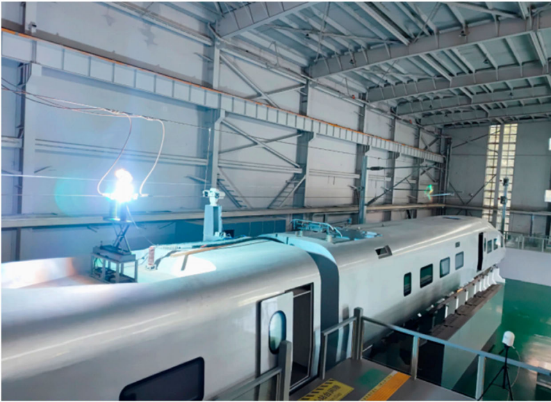
Figure 10. Arc phenomenon between the CL and pantograph. Source(s): Yang et al. (2024b)
