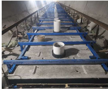
Plate 1. The steel limiting beams
