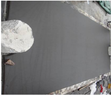
Photo of CA mortar after removing slab
