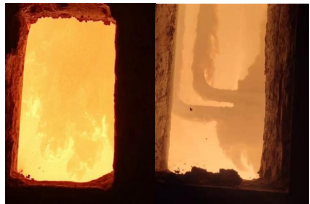
图 4 锅炉供热季结渣示意 Fig.4 Schematic diagram of boiler slagging during heating season
