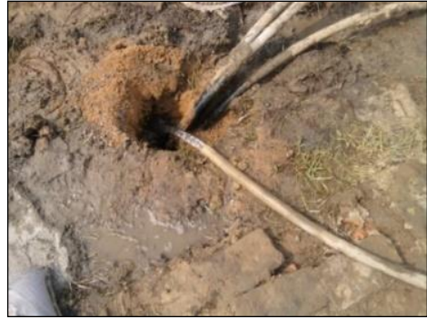
图4 钻孔现场回填 Fig.4 Backfilling at drill hole site
