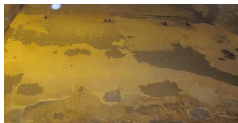
图 6 炉膛前后墙 FGR 喷口布置和前墙 FGR 喷口现场照片 Fig.6 FGR ports arrangement on the furnace front and rear walls and the in-situ picture of the front wall FGR ports
