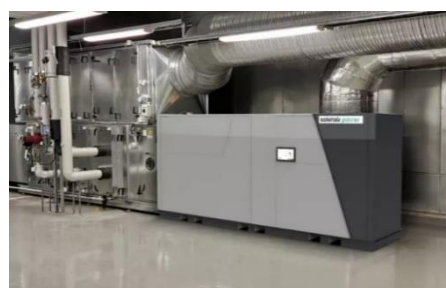
图 5 Soletair Power 的 HVAC-DAC 集成系统 Fig.5 The HVAC-DAC integrated system of Soletair Power
