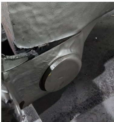
图 1 限位卡块磨损断裂 Fig.1 Limit block is worn and fractured
