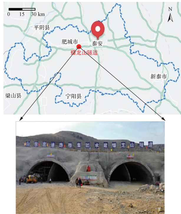
图4 隧道地理位置和入口外观 Fig. 4 Tunnel location and entrance appearance
