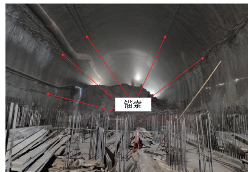
(c) 拆除临时支撑
