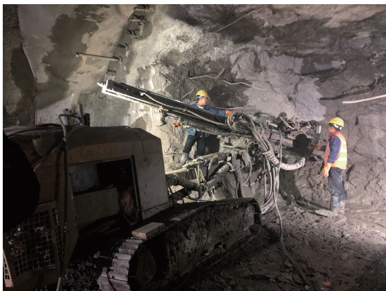
(a) 掌子面打设试验桩
