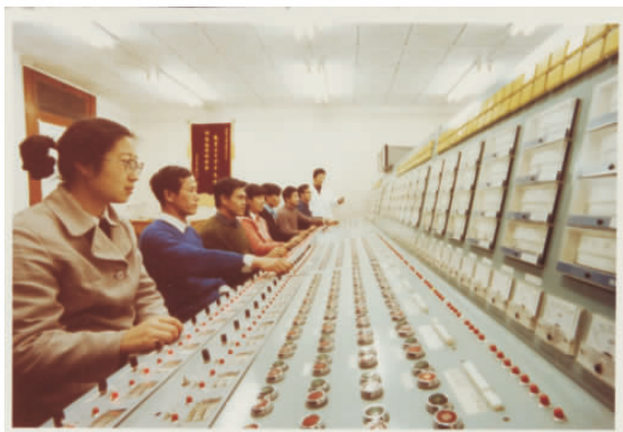
图 1 清华大学研制的我国首台火电仿真系统 Fig. 1 The first power plant simulation system in China, developed by Tsinghua University
