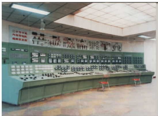
图 2 清华大学研制的我国首台全范围仿真机控制室 Fig. 2 Control room of the first full-scale simulator in China, developed by Tsinghua University
