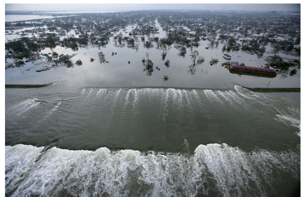
图7 2005年Katrina飓风导致决堤,大量洪水涌入市区 Fig. 7 Hurricane Katrina destroyed floodwall, floodwater poured into city of New Orleans
