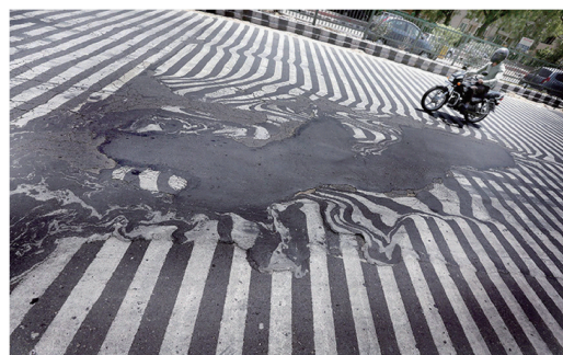
图 13 2015 年 5 月印度新德里高温引起的路面标示变形 Fig. 13 Distorted road markings as the asphalt melted due to high temperatures in New Delhi
