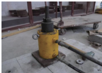
图4 实施拉拔 Fig. 4 Implementation of pull-out
