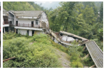
图2 虹口八角庙部队 培训楼遭破坏 Fig. 2 Collapsed training building in Bajiaomiao, Hongkou
