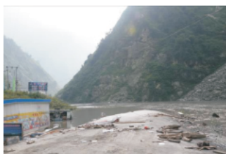
图 9 “8.13”强降雨形成的堰塞湖(K7+000) Fig. 9 Dammed lake caused by heavy rains on August 13, 2010
