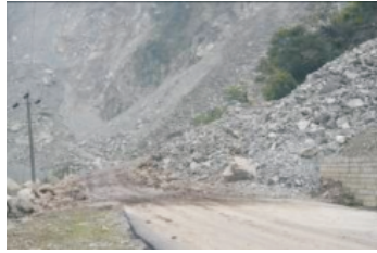
图 13 崩塌堆积物掩埋公路 Fig. 13 Provincial road S303 buried by collapse accumulation
