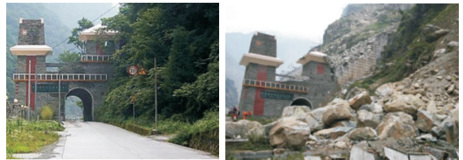
图 14 S303 线卧龙山门震前(a)、震后(b)的对比 Fig. 14 Comparison of Wolongshan gate in provincial road S303 before (a) and after (b) the earthquake
