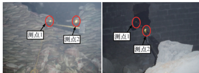
(a) 以沙包为支撑 (a) Supported by sandbags (b) 以水泥砖墙为支撑 (b) Supported by cement bricks
