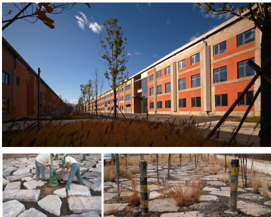
图 38 建筑拆除构件二次利用于园区景观建设 Fig. 38 Secondary utilization of demolished building components for park landscape construction
