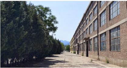
图 11 厂房原门窗 Fig. 11 Original doors and windows of the factory building
