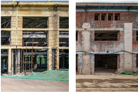
图 29 砖墙构造柱与圈梁加固现场 Fig. 29 Strengthening construction site of constructional columns and ring beams for brick walls
