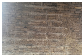
(a) 拱券嵌筋加固修缮后
