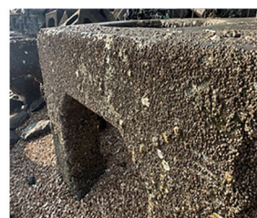
(b) Barnacles and oysters extensively covering a breakwater in Tianjin
