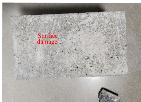
(b) Surface erosion and deterioration of concrete (600 freeze-thaw cycles)
