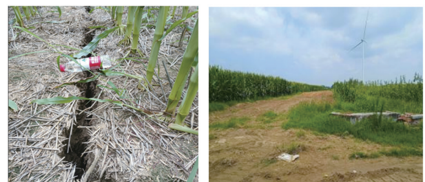
(a) 侧移导致地裂缝
