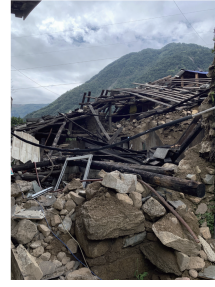
图 4 以石、土作为主要承重构件的房屋 Fig. 4 A building with stone and soil as the main load-bearing components
