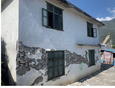
图 3 以砖石为主要承重构件的房屋 Fig. 3 A building with masonry as the main load-bearing components
