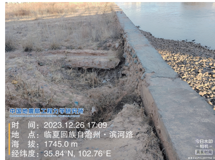
图 10 北侧拦河堤外闪(闫培雷摄) Fig. 10 Moved outside of the north side of the barrage (Photo by YAN Peilei)
