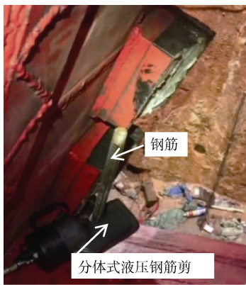
图 5 仓内剪切钢筋示意 Figure 5 Schematic of cutting steel bars
