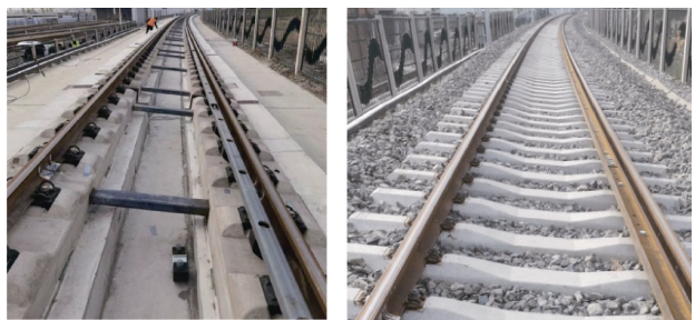
图6 梯形轨枕无砟轨道与普通有砟轨道现场 Figure 6 Site photos of ladder-sleeper ballastless track and ordinary ballasted track
