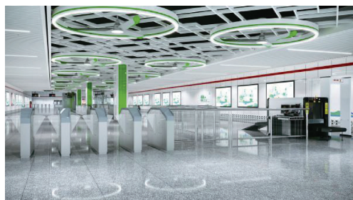
图 2 永磁仿自然风风扇布置图 Figure 2 Layout of Permanent Magnet Imitation Natural Wind Fan
