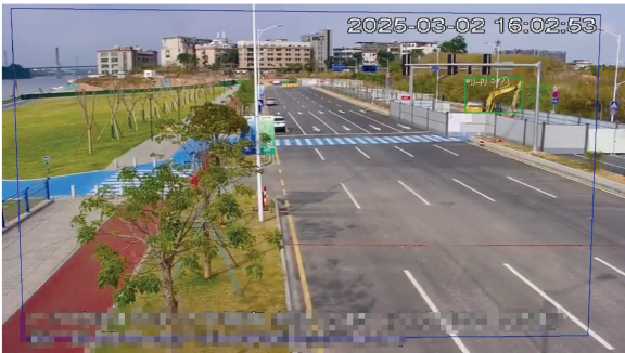
图 5 地铁保护区视频智能巡检系统应用测试效果 Figure 5 Application effect of video intelligent inspection system in subway protection area
