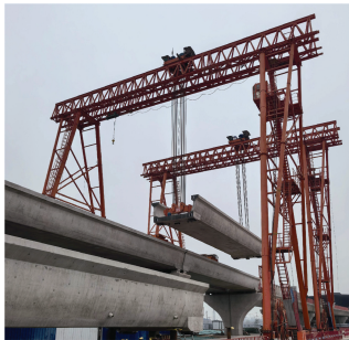
图3 正在架设中的U梁 Figure 3 U-beams being erected
