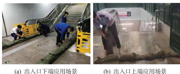
图 1 防汛沙袋 Figure 1 Flood control sandbags
