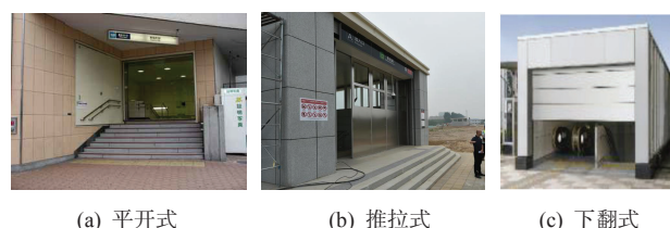
图 3 挡水门 Figure 3 Water stop door
