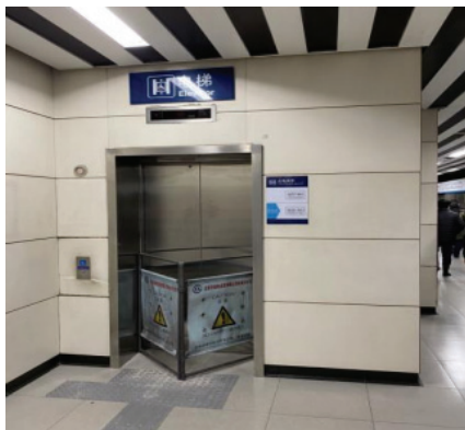
图11 电梯井围挡应急处置示例 Figure 11 Example of emergency response to elevator shaft enclosure
