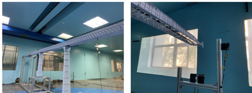
(b) 钢箱梁和钢导梁局部构造 (b) Details of the box girder and guide girder
