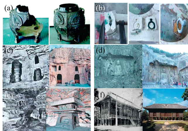
Fig. 10. (a) Condition of primeval an ancient small-mouthed wine vessel before and after restoration. (b) Repair the cover button with 815 epoxy resin. (c) Comparison before (left) and after (right) restoration of Grottoes 1 and 2 in Yungang Grottoes. (d) Comparison before (left) and after (right) restoration of "Epoxy resin grouting technology for surrounding rock reinforcement" at the Great Shrine of Fengxian Temple. (e) Comparison before (left) and after (right) restoration of the central tower column in Cave 1 of Yungang Grottoes. (f) Comparison before (left) and after (right) restoration of Horyuji.
