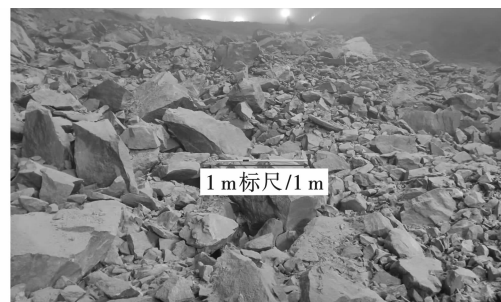
(b) 地下厂房Ⅲ层 (b) The third floor of the underground powerhouse
