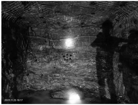
图2 井下小断面开挖融合延时起爆网路现场 Fig. 2 Fusion delay initiation network for small-section excavation
