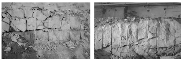
(a) 上游预裂爆破效果 (a) Upstream pre-splitting and blasting effect (b) 下游预裂爆破效果 (b) Downstream pre-splitting and blasting effect
