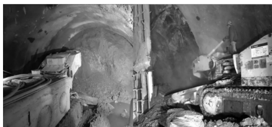
(a) 上断面机械法施工 (a) Mechanical construction of the upper bench
