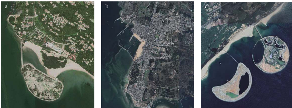
Fig. 2. Schematic diagram of coastal defences. Longitudinal structure (a), perpendicular structure (b), detached structure (c).
